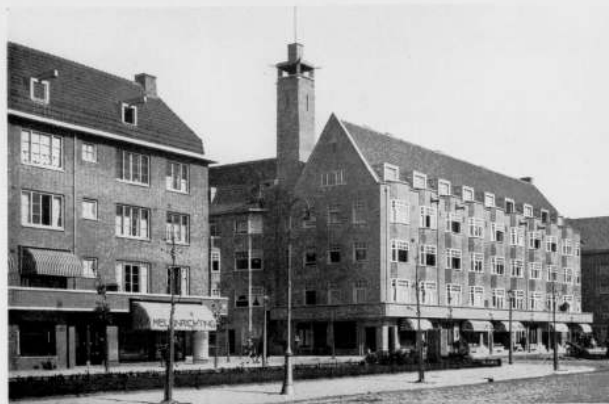
ARCHITECT G. J. RUTGERS, RECHTER BOUWBLOK; ARCHITECT CH. DEKKER, LINKER BOUWBLOK
